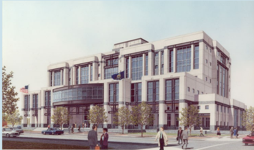
Federal Courthouse Kansas City, Kansas
